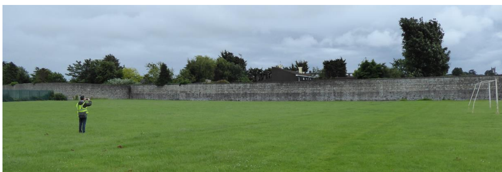
Figure 17.15 – Internal face of Perimeter Wall to west of the Site
