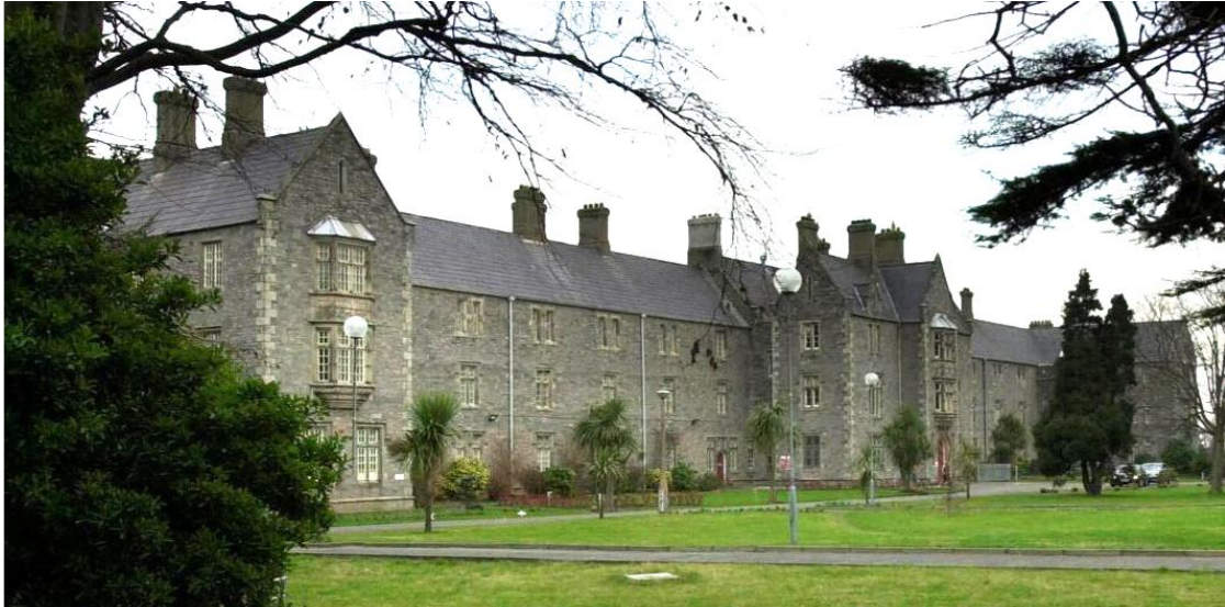
Figure 17.11 – Main Hospital Building
