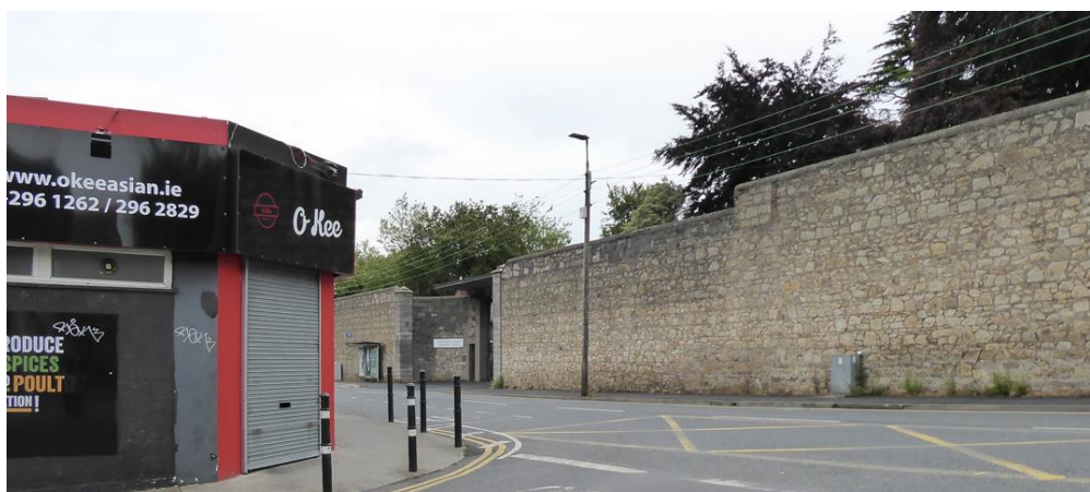
Figure 17.14 – Perimeter Wall and Entrance on Dundrum Road
